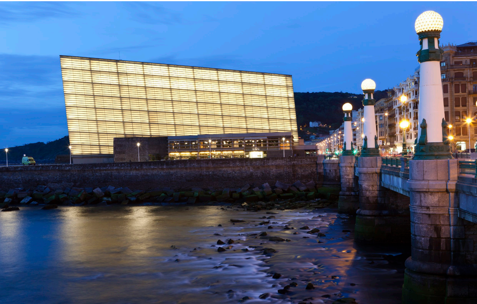
▲ CONGRESS HALL AND KURSAAL AUDITORIUM DONOSTIA-SAN SEBASTIÁN
